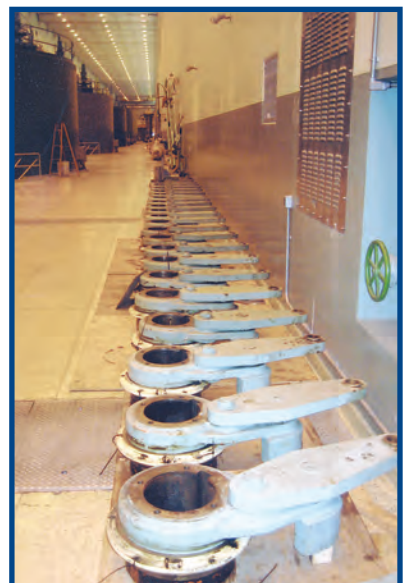
WICKET GATE READY FOR REBUILD
