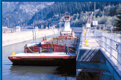
LOCK GATES & MOORING BITTS
