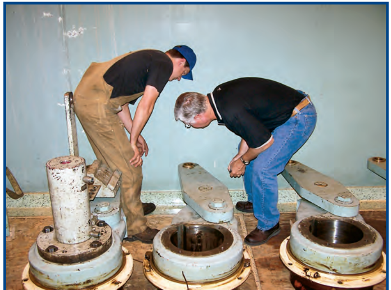
MARSHAL WADDINGTON (USACE) AND STEVE PHILLIPS (CIP) INSPECTING WICKET GATE LINKAGE.
