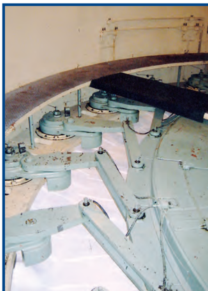
OPERATING RING WITH LINKAGE TO WICKET GATES
