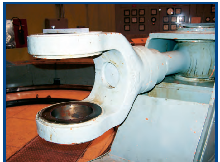
GATE SERVO OPERATING RING CONNECTION, PIN REMOVED
